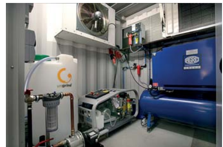
Separate compartment with Compressors
